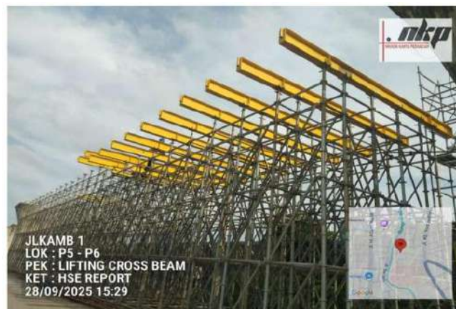
Install shoring dan Cross beam Span P6-P5
